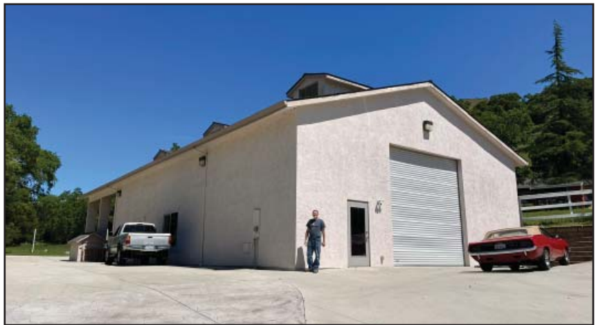
This beautiful workshop is not only spacious and well-lit, it's also remarkably cool during hot weather, and easy to heat during the winter
