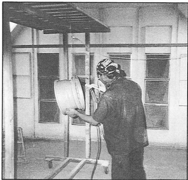
Each wheel is sprayed with powder paint, then wheeled into a giant oven where the finish is baked on and the wheel is annealed again (all the wheels were treated at the same time; these photos were taken merely to illustrate the process)
