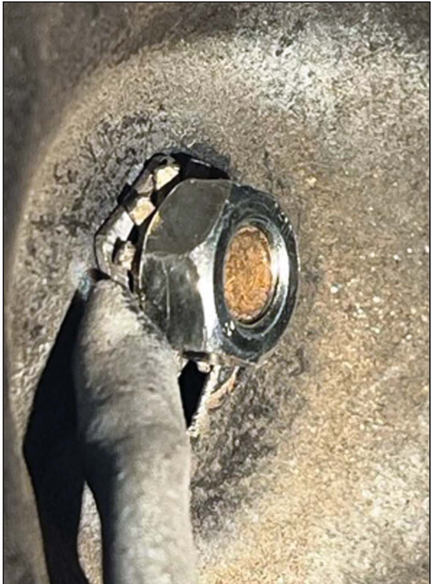
The star washer was installed in between the nut and the eyelet on the factory ground wire, and suddenly everything started working properly once more
