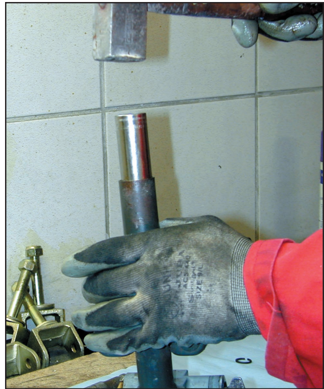
A deep socket is used as the drive tool, to drive the new bearing into the steering column tube until it comes to rest against the stops
